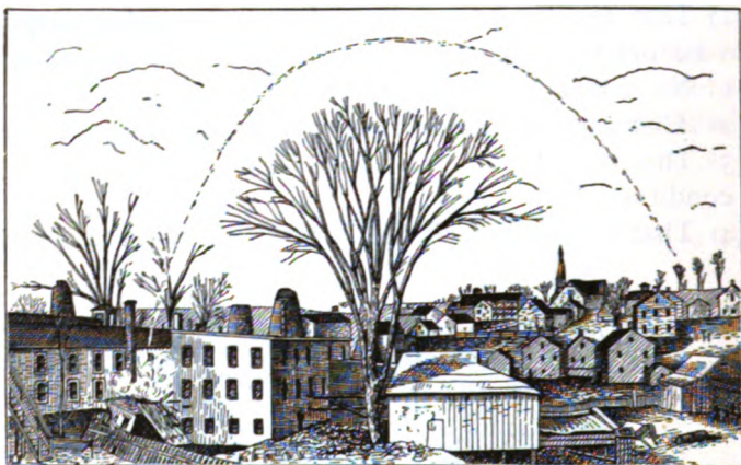
FIG. 172.—EXPLOSION OF AN UPRIGHT BOILER.
